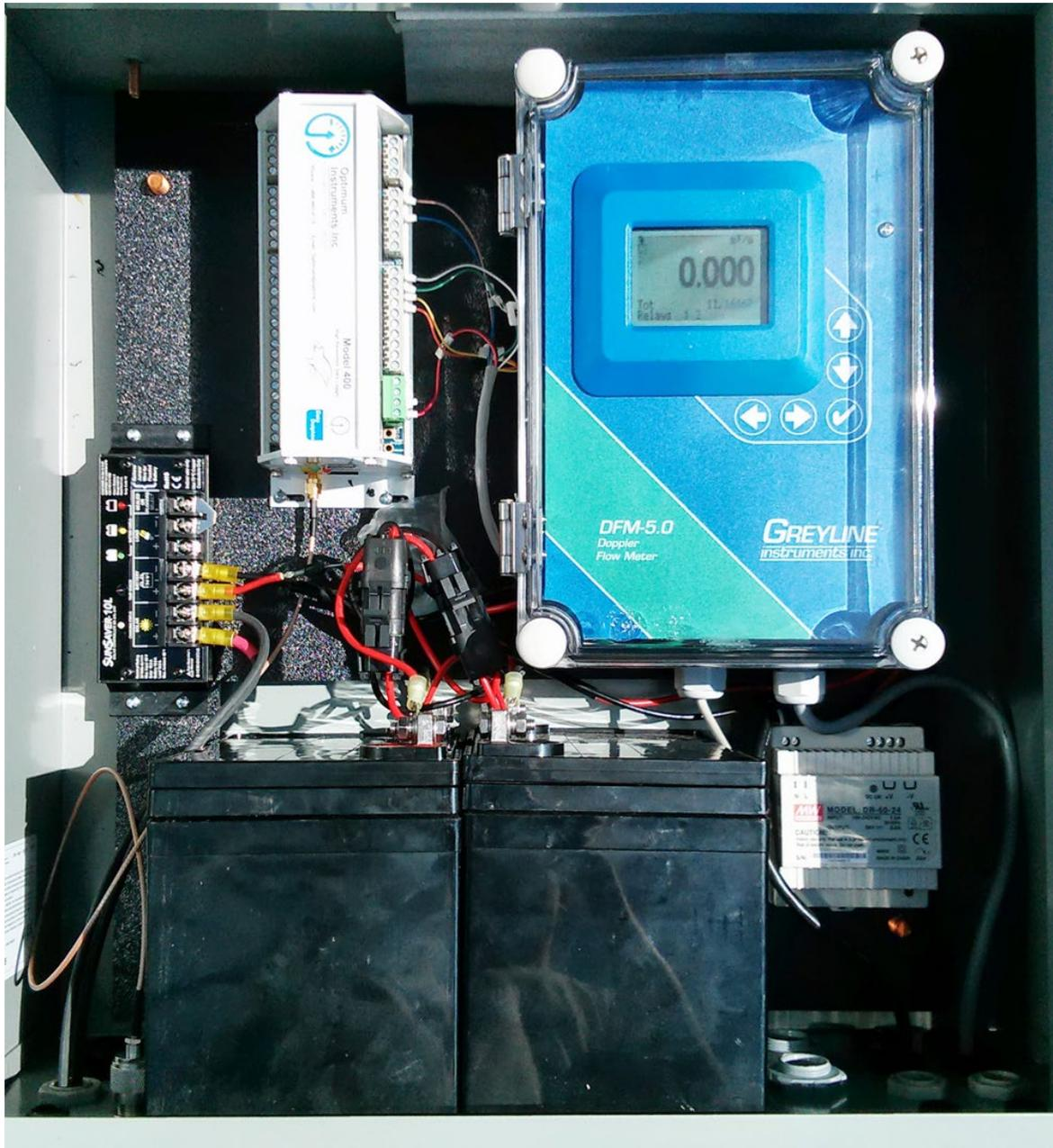
If your system is 24V the batteries will have connectors to mate to internal wiring harnesses. There is no worry about which connector goes to which side as they can mate correctly either way. To install your batteries insert the first one with the terminals on the left side and slide it into the right position. Then drop in the next battery with the terminals to the right beside the first one.
